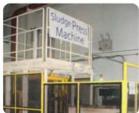
PUTTING INTO SLUDGE PRESS MACHINE
