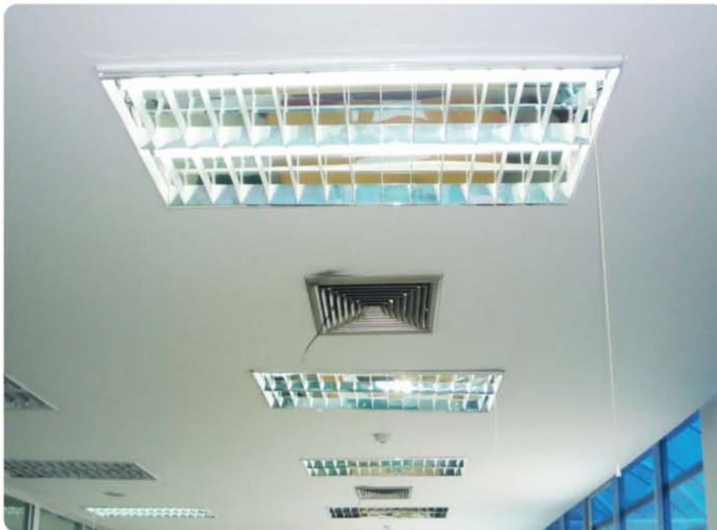
SAVE ENERGY BY USING MANUAL SWITCH
