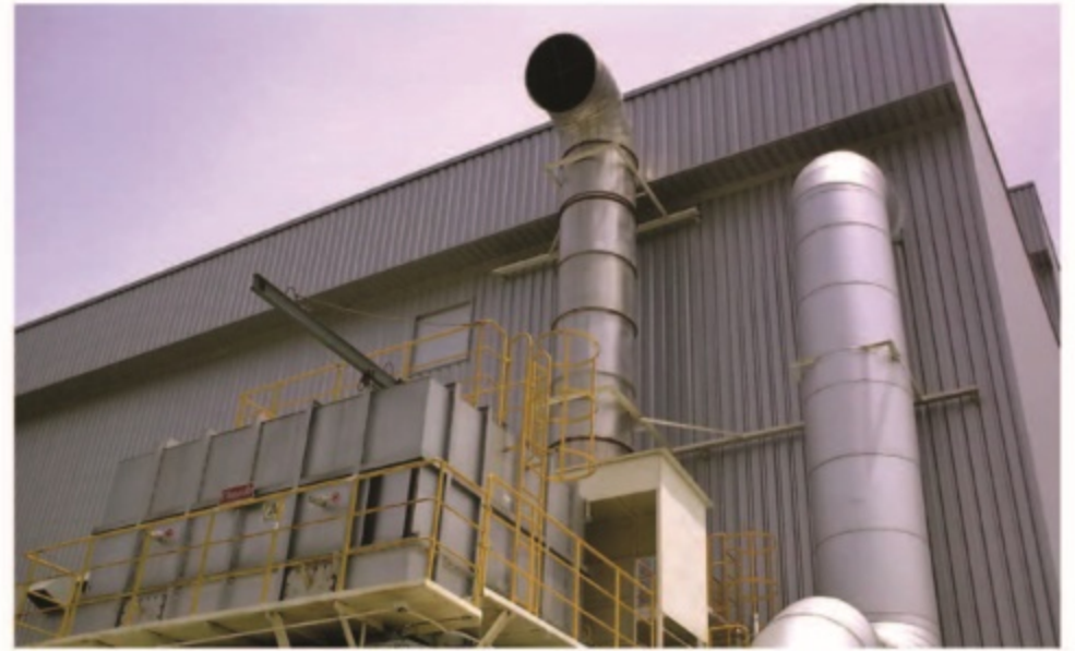
RTO machine: Regenerative Thermal Oxidizer for VOC (Volatile Organic Compound) treatment
