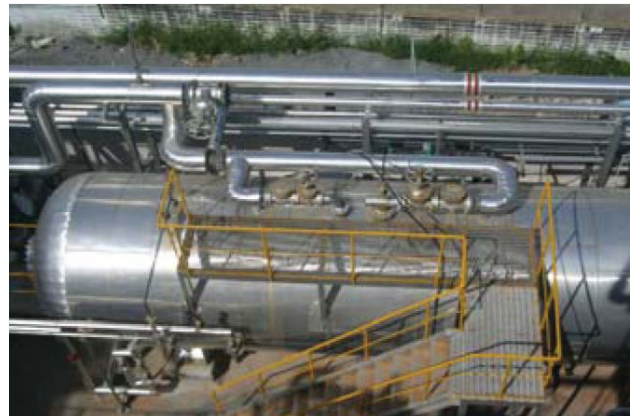
Boiler for steam production using heat from waste incineration
