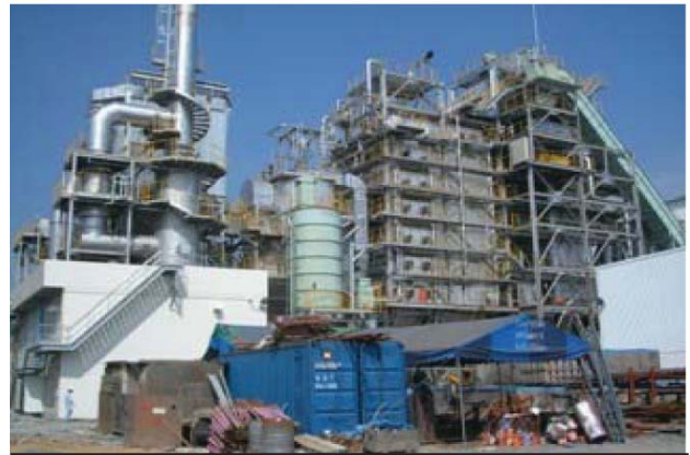
Waste incinerator with steam production
